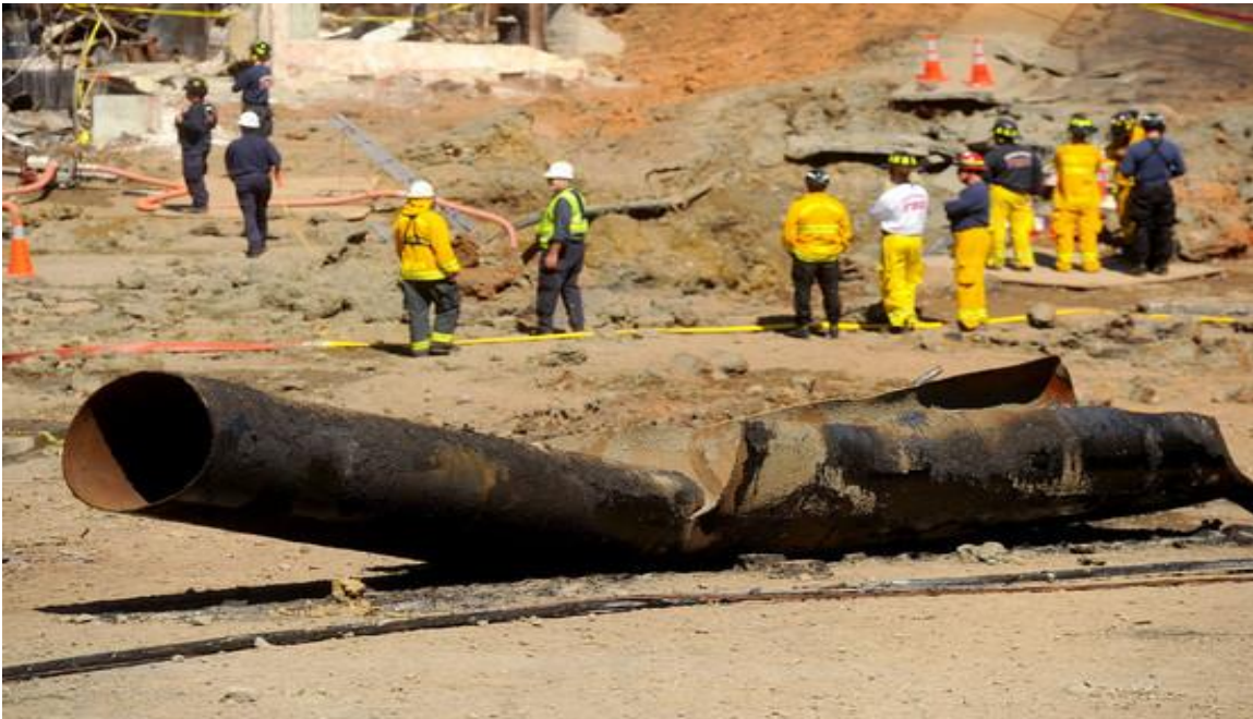
Figure 4 shows the result of a SCC crack growth failure.
